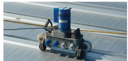
Butler's exclusive Roof Runner® completes the industry's only field-formed 360-degree Pittsburgh double-lock seam.
